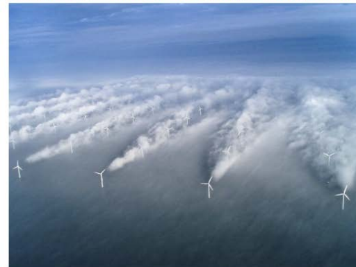
Figure 2. Turbulent wakes downstream of windmills. These wakes decrease the energy output of the windmill park. The wakes are formed when water vaporizes in the low pressure region downwind of the windmills. ( https://img.dk/artikel/eons-nye-vindmoller-stjaeler-vind-fra-dong-97227 )
